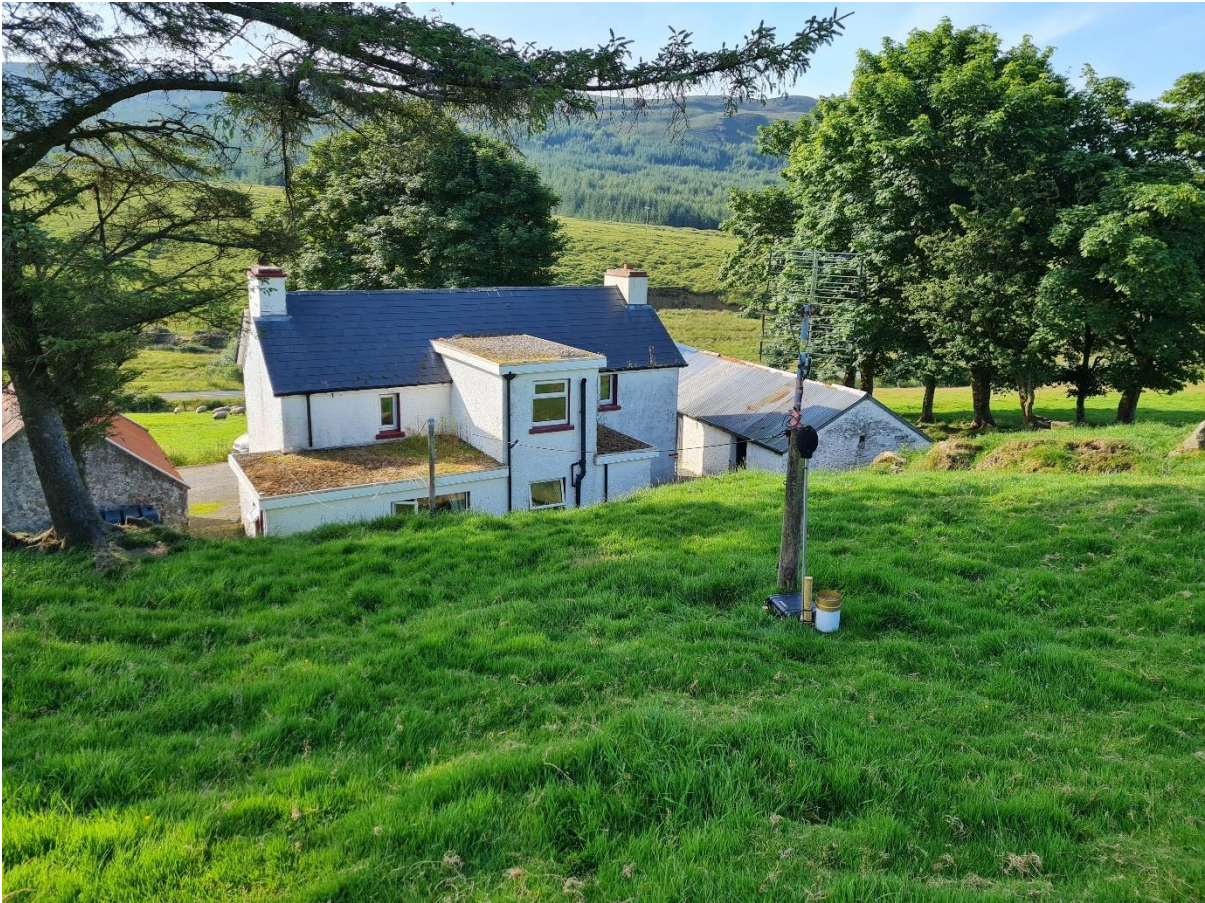
Figure 12-8: Noise Monitoring Installation – NML-6
